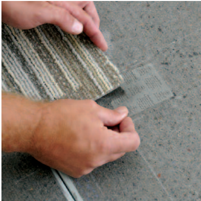
TacTiles connectors are adhered to the corners of InterfaceFLOR carpet tiles.
