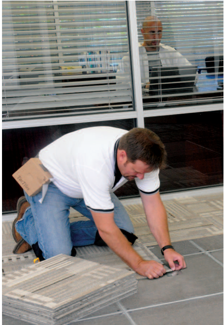
You can install InterfaceFLOR carpet tile with TacTiles connectors almost anywhere at anytime.
