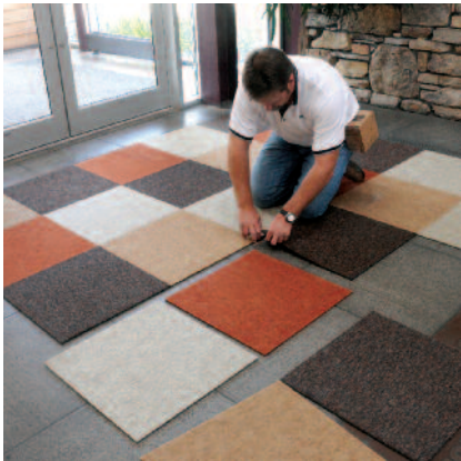
Use TacTiles connectors to install area rugs in addition to wall-to-wall installations.
