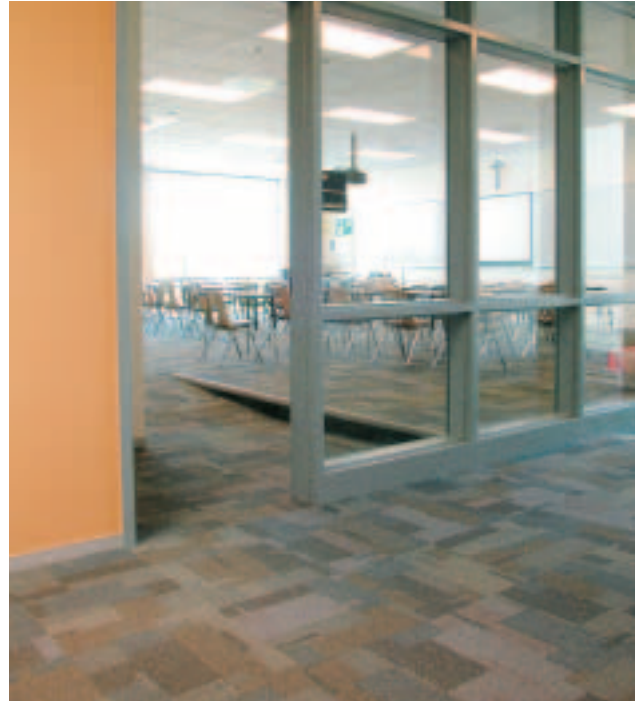
Interface carpet helps to dampen sound and improve acoustics in classrooms.
