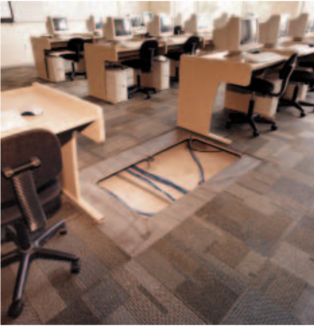
In the Strake computer labs, Entropy was used on top of Interface's TecCrete access floor system.
