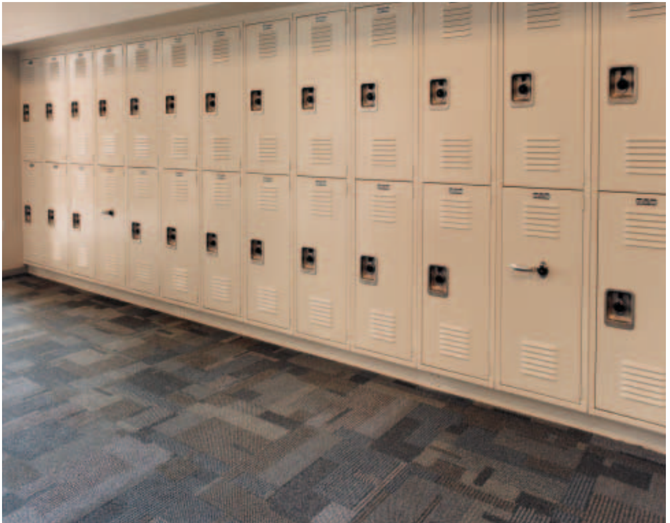
Even after a year of heavy traffic, the Entropy carpet in this locker area still looks new.
